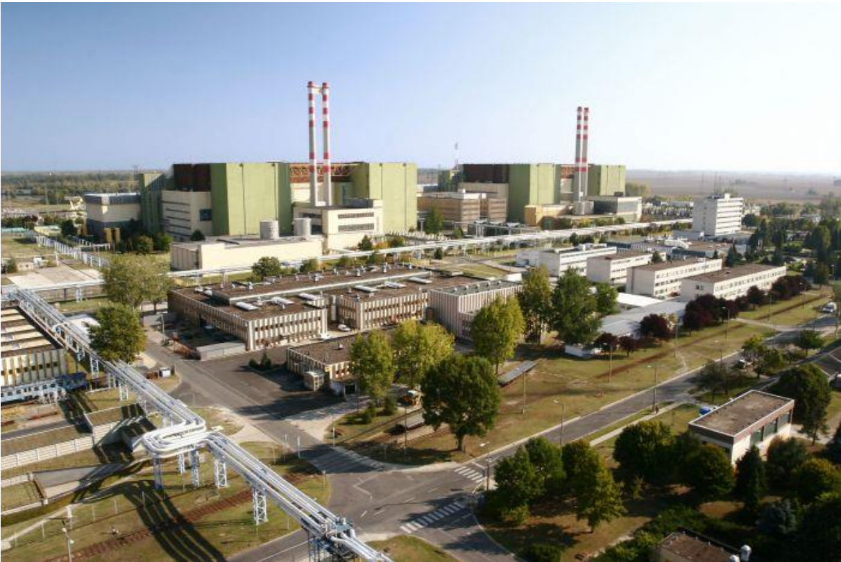
The main buildings of the Paks NPP (source: [1])
